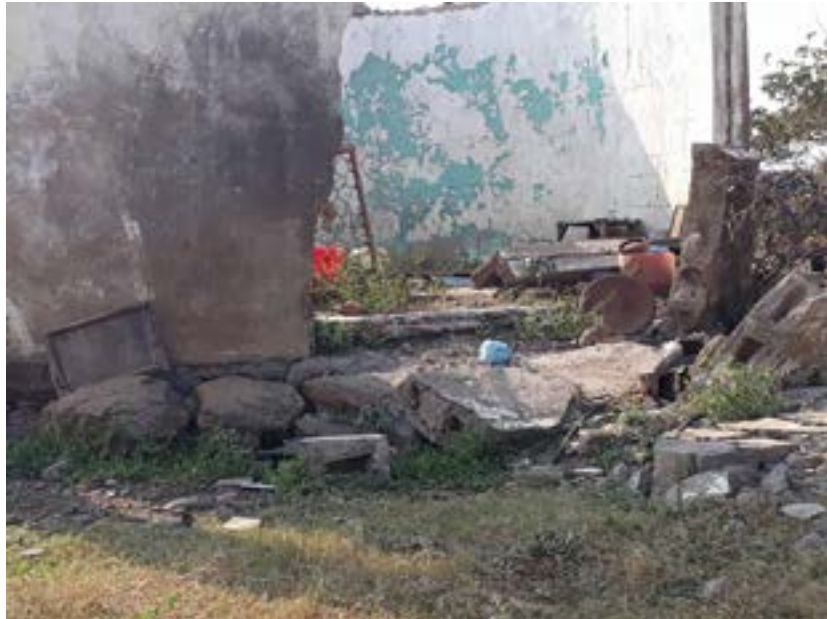
A collapsed structure in Bab Mtshali's yard, the damage was caused by the constant blasting coming from Somkhele Mine.
